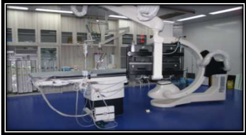
Gb. Instalasi Diagnostik Intervensi Kardiovaskuler
